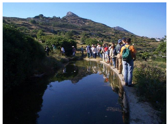
Figure 15. Result of enrichment of the aquifer by the small dams in Apeiranthos, Naxos, at 650 m altitude, 7-15-2000. Source: I. N. Hatzopoulos.
