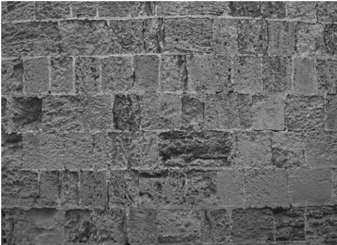
Fig. 13. The preservation state of the building stone at "Position 5" is adequate. Decay can be detected on the external surface of the stone.
