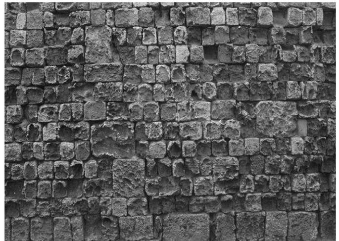
**Fig. 12.** Building stone preservation state at “Position 2”. Severe weathering followed by granular disintegration and material loss is presented.
